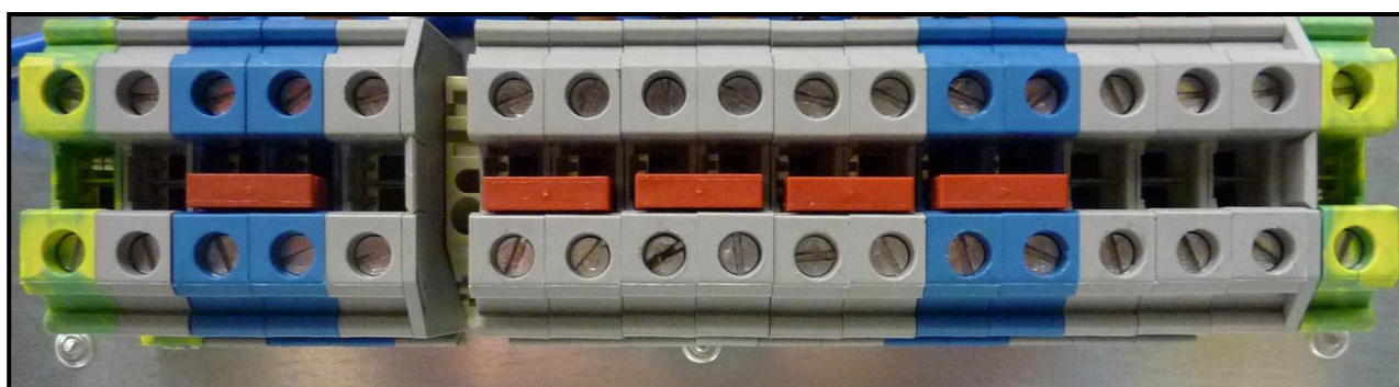
Figure 2.2 10-15-20-30 kVA Cable Connection
