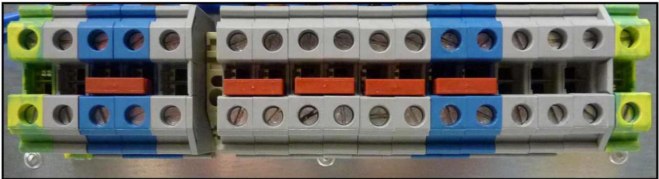
Figure 2.2 5-10-15 kVA Cable Connection
