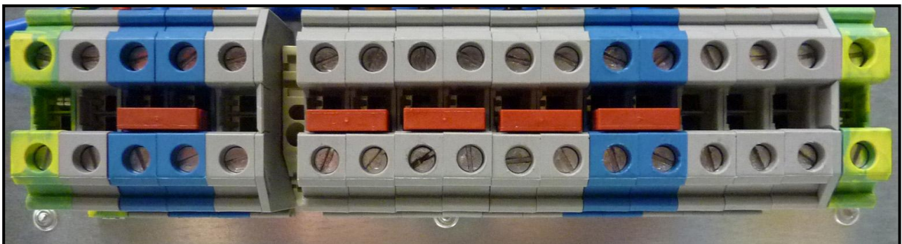
Figure 2.2 10-15-20-30 kVA Cable Connection
